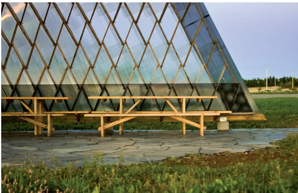
TOP AS PART OF DALHOUSIE'S COASTAL STUDIO, A GROUP OF ARCHITECTURE STUDENTS DESIGNED AND BUILT LAMELLA, A HELICAL PERGOLA THAT IS AN ELEGANT AND SIMPLE EXPRESSION OF FORM. ABOVE A DETAILED VIEW OF LAMELLA AS IT MEETS THE GROUND.
